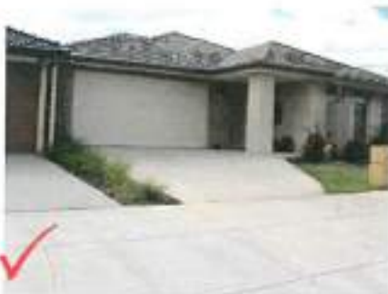
Example of a compliant design for a garage, with a red checkmark to show it is a desirable outcome.
