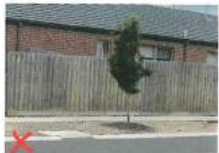
Example of non compliant timber paling fence without capping and exposed posts.
