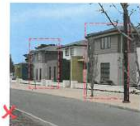
Example of two dwellings with identical facades. This is not permitted.
