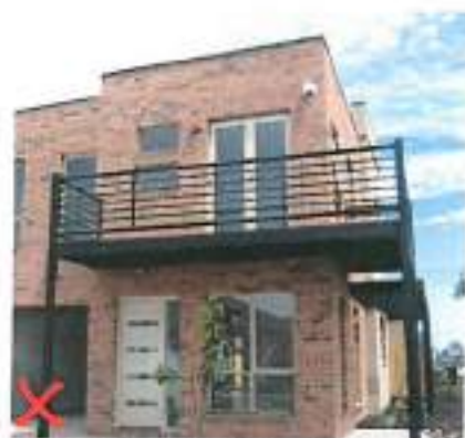
Example of a uniform brick facade, no differentiating materials.
