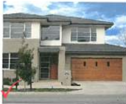
Example of a two-storey dwelling with a garage, represented with a red checkmark to denote a good example.
