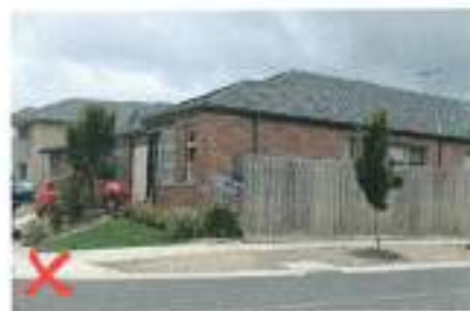
Example of non-compliance with the 5m setback from the rear lot boundary.
