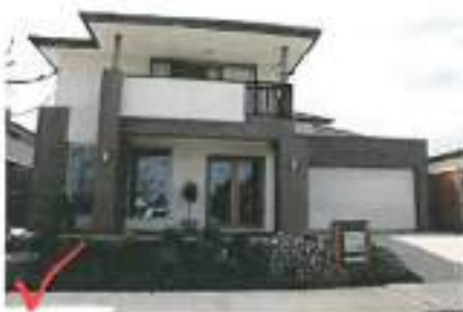
Double-storey dwellings which incorporate a minimum width 1.5m covered veranda/ balcony to the first floor for at least 40% of the home width do not require the setback between the front wall and garage.
