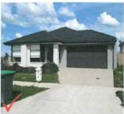
Garage setback from front boundary must be behind facade of the house.
