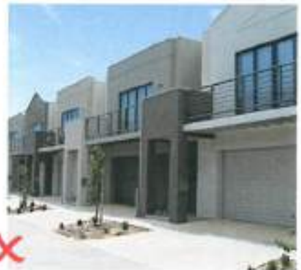
Example of non compliant treatment, no setback.
