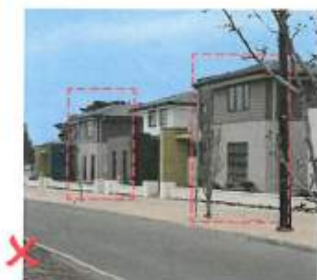
Example of non-compliant facade, identified by a red 'X' in the image.
